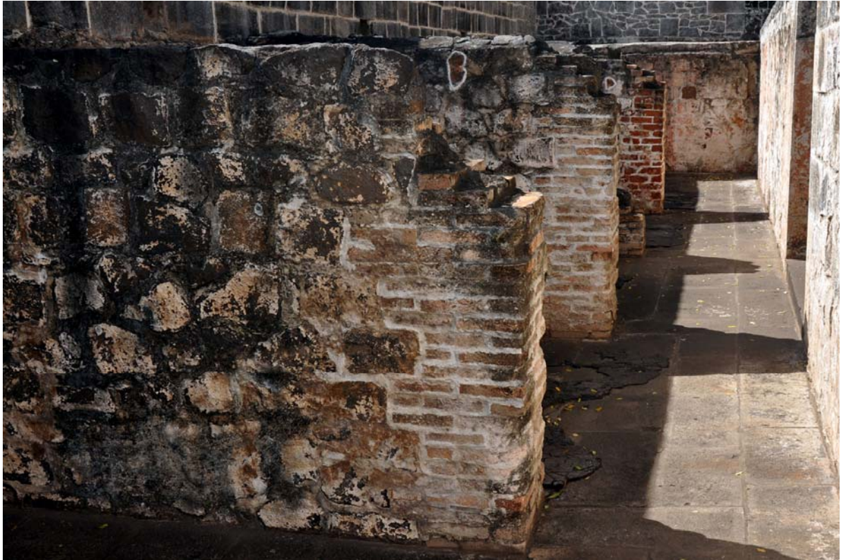
Figure 6. Yellow imported fire bricks and larger Mauritian red bricks recycled in modifications to the Sector P Privies; note also the bitumen covering basalt flagstones. (ph 1174)
