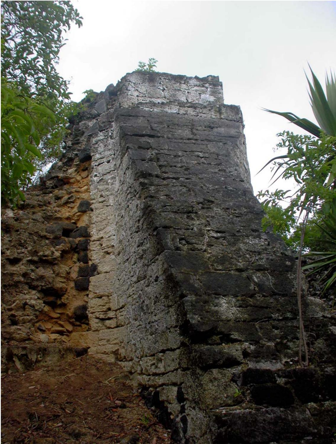
*Kiln I Buttness 2 is also the end of the spiral staircase. The buttness itself is completely preserved and it can be seen from this image that it is generally butted against the basalt facing of the furnace although the two have occasionally been bonded together – showing that the buttness and the spiral staircase were an integral part of the original design rather than a later addition. (ma03jv0305)*
