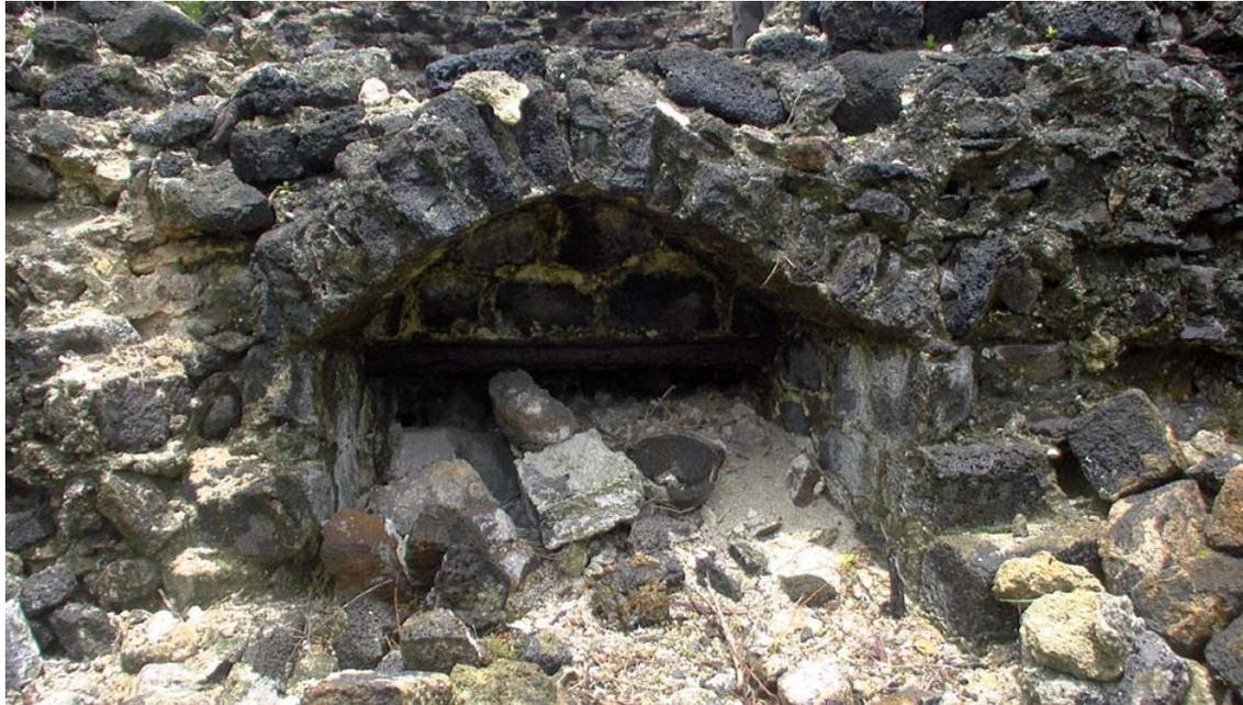
*The splayed draw hole of Kiln 2. The slightly pointed arch is constructed of uncut basalt stones set on edge. The internal iron lintel is heavily corroded. (ma03jv0212)*
