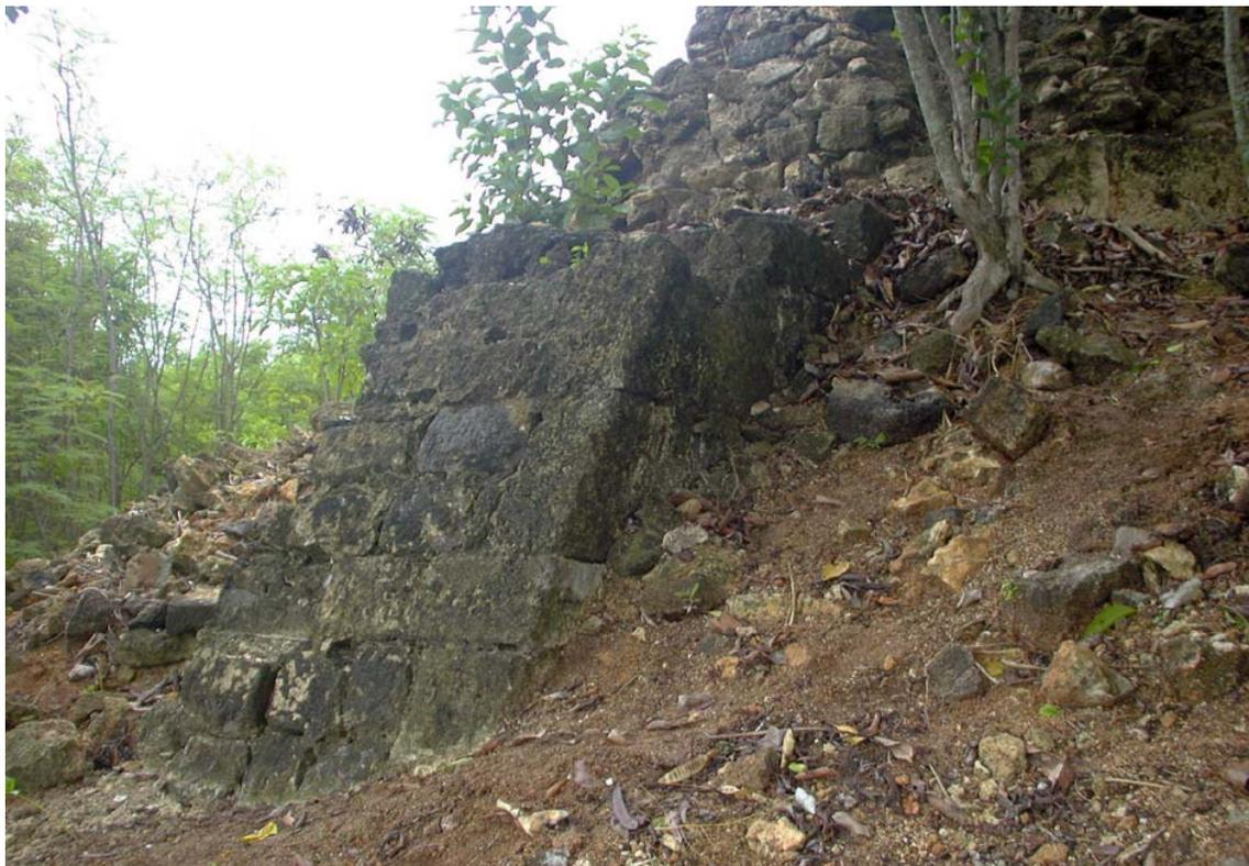
*Kiln I. The first buttress is constructed of coral and is bonded into the furnace wall. The 1922 photograph shows that it did not extend to the top of the furnace but ended on a level with the tops of the recessed features on either side. The width is 1.15m. (ma03jv0311)*
