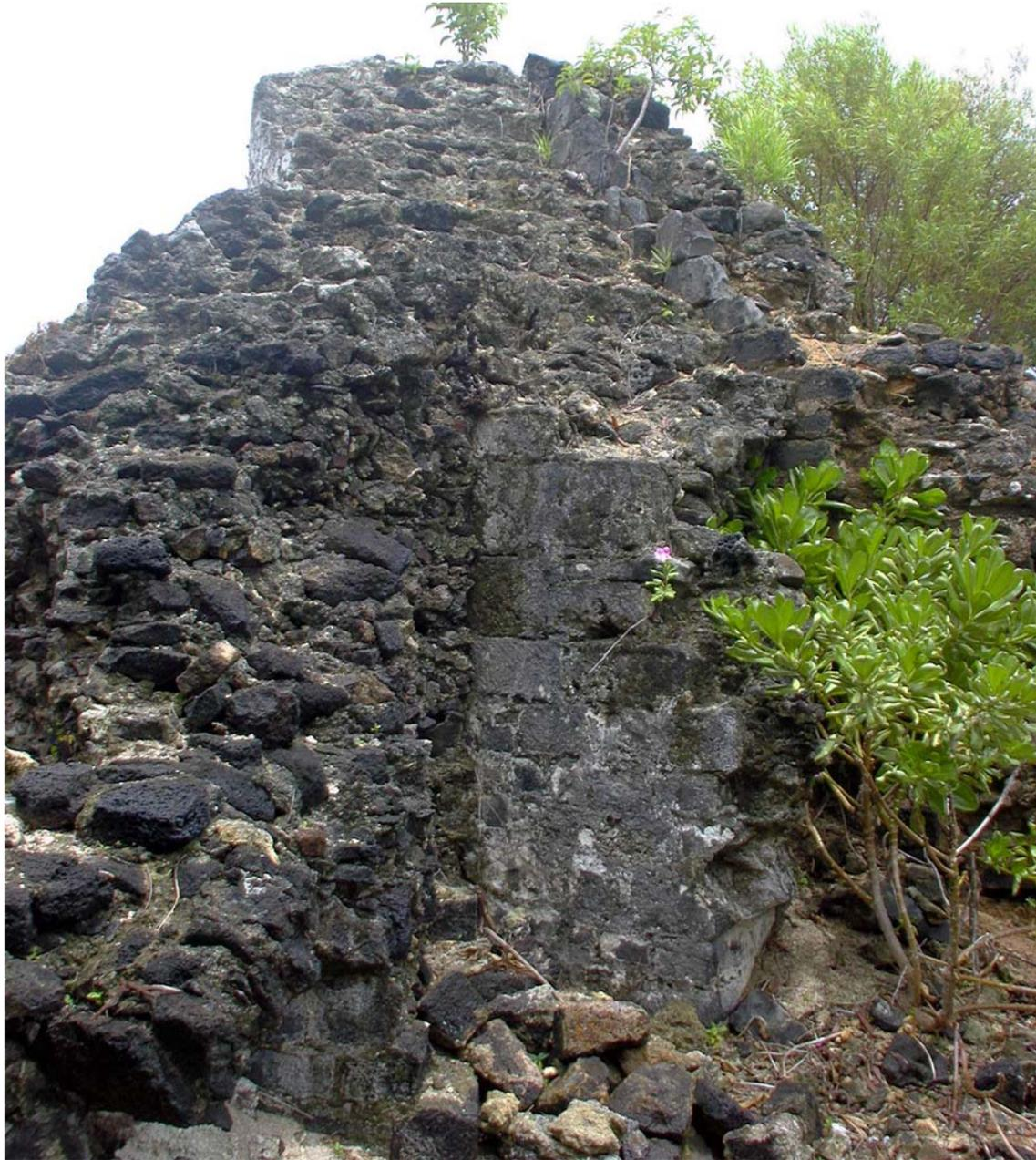
*The wall of Kiln 2 butts against the stairs of Kiln 1. The steps and lining of Kiln 2 have been robbed. The basalt facing of Kiln 1 is preserved behind the staircase from which it protrudes. The springing of the basalt arch beneath the stairs can be made out to the right of centre at the bottom of the picture. (ma03jv0211)*
