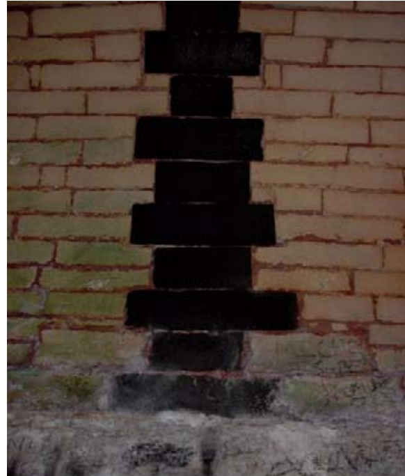
Details of the barrel vaulted ceiling showing the two sides of a basalt arch, the cutting of the fossilised coral blocks to fit and support the basalt during construction, and the use of waterproof lime mortar mixed with crushed brick for the vault. Some of the graffiti carved into the coral by British soldiers in the 1840s are visible. The walls are rendered below the springing. (01jv0601 & 0602)
