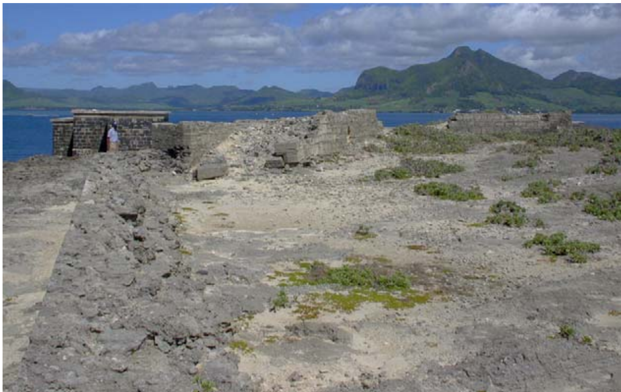
The junction Wall A2 and A3 showing how the upper part and inside face of A3 was demolished up to the now the ruinous ramp and platform supported by Wall D. The roughly levelled area behind the Lower Battery can also be seen. (02jv1904)
