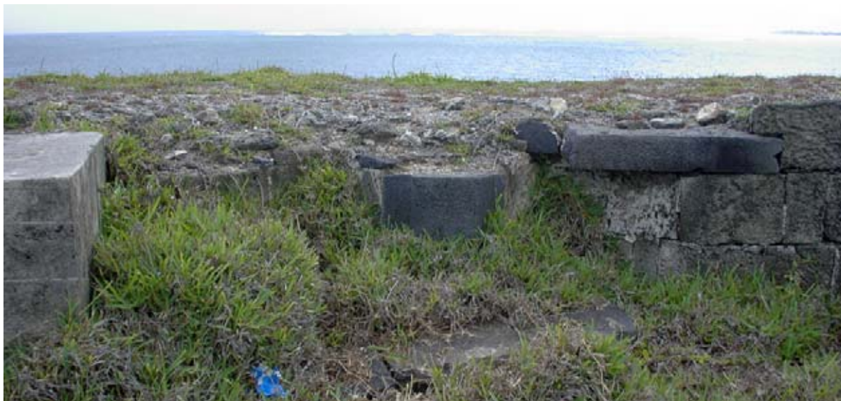
One of the emplacements with triangular niches divided and capped by basalt ashlar. Note the displaced stones in front and WW II concrete at left. (02jv0409).
