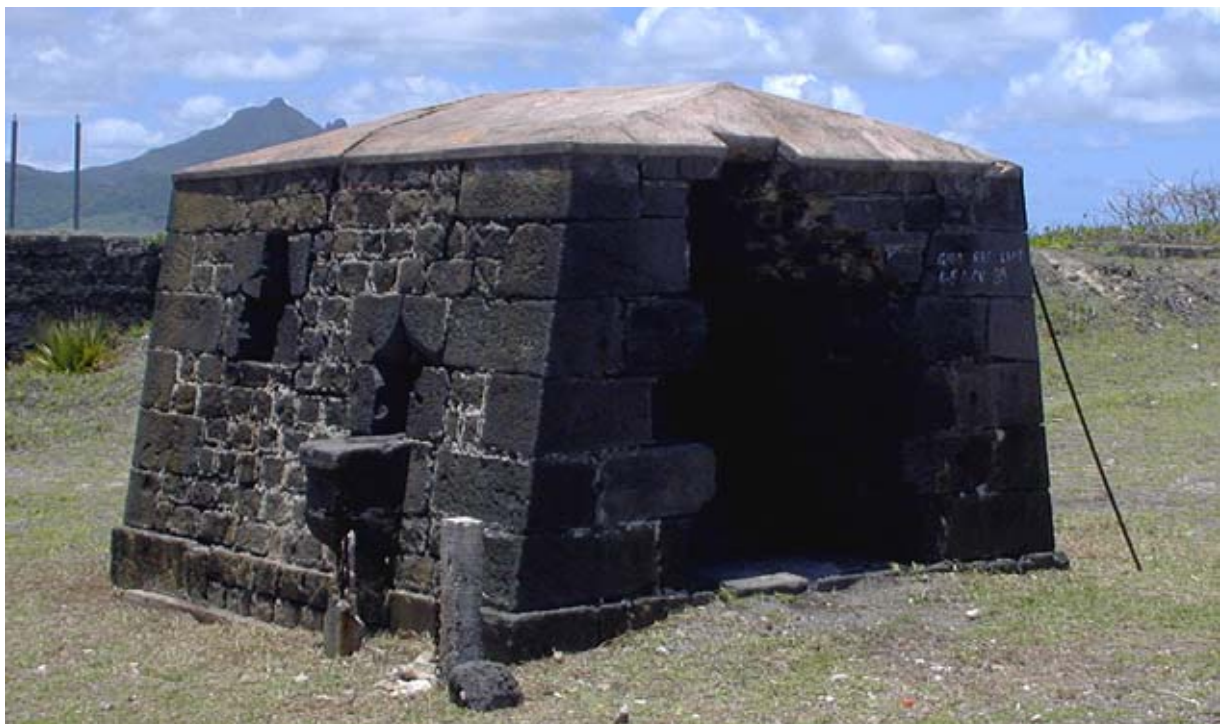
The west side of the Shot Furnace showing the cantilevered receptacle and the higher opening behind into which cannon shot was placed. The form of the roof can be clearly seen. The concrete posts are modern. (02jv1118)
