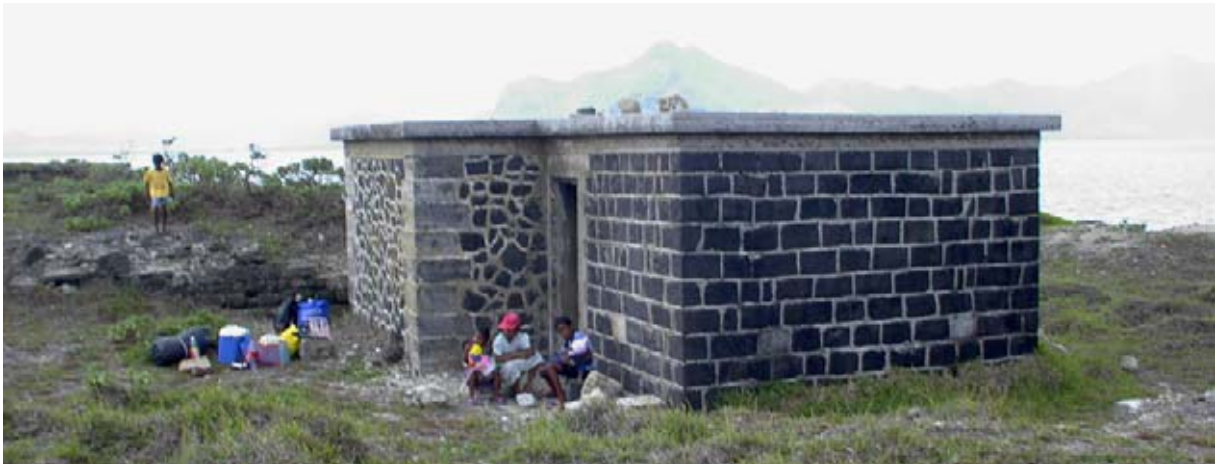
The original phase of the Central Building comprised a single room built of basalt ashlar with concrete tie blocks. The addition was uncoursed with pre-cast quoins. (02cn0423)
