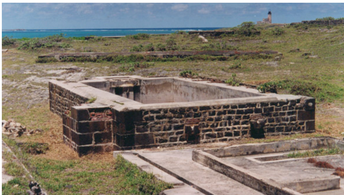
The Cistern or Tank (Structure 4) which was, as can be seen from the bevelled cement surround on the top, reused in WW II. Part of the Cook House (Structure 6) is in the foreground and the platform for Structure 17 is at centre. (02cn0401)
