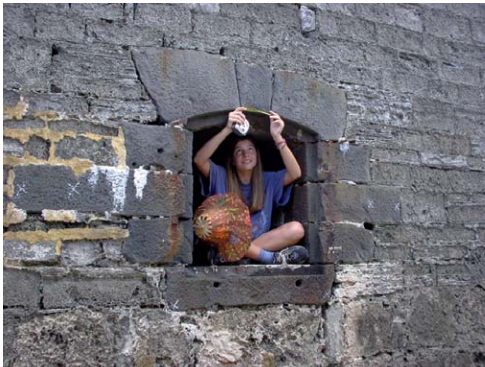
Measuring the window. (02jv0704)
