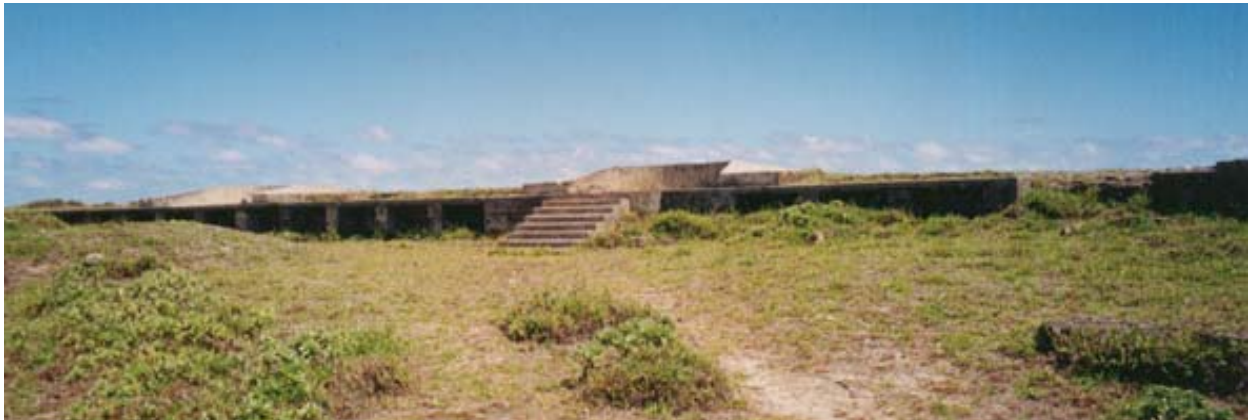
The WW II Upper Battery with the emplacements for two large guns and the shell cabins which were constructed behind and on top of the earlier French work. (02cn0420)
