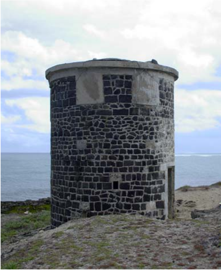
The upper windows, blocked in WW II, the construction stages and the original precast tie blocks. (02jv0415)
