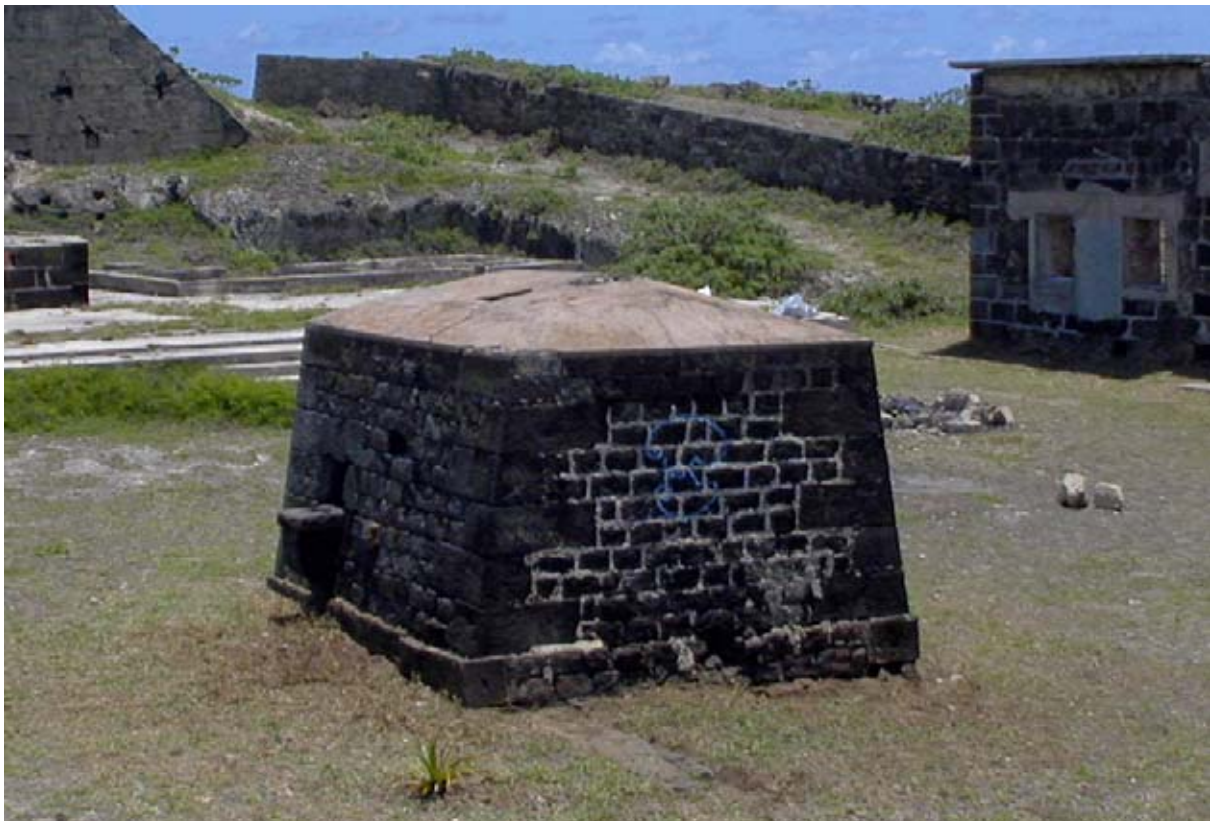
The Shot Furnace from the north-west with an earlier wall foundation projecting from the back wall at bottom centre. (02jv1207)
