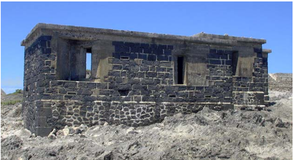
The Western, Searchlight, Building (Structure 12) from the west showing WW II modifications to the original windows. (02jv0902)
