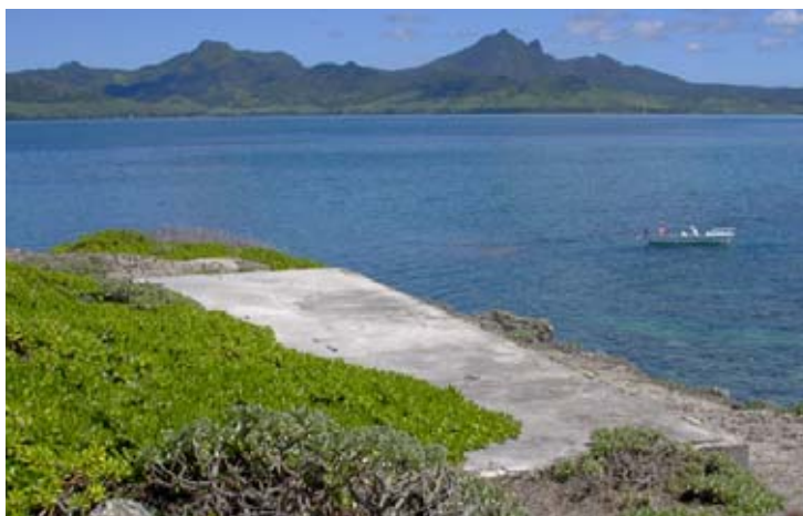
Structure 29 from the north. (02jv2214)
