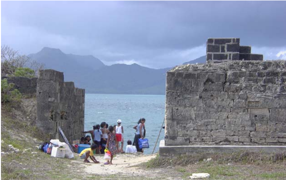
The landing Point with the west end of Wall H, at right, showing modern concrete underpinning and the flag emplacement, Structure 31, above. (02jv0410)
