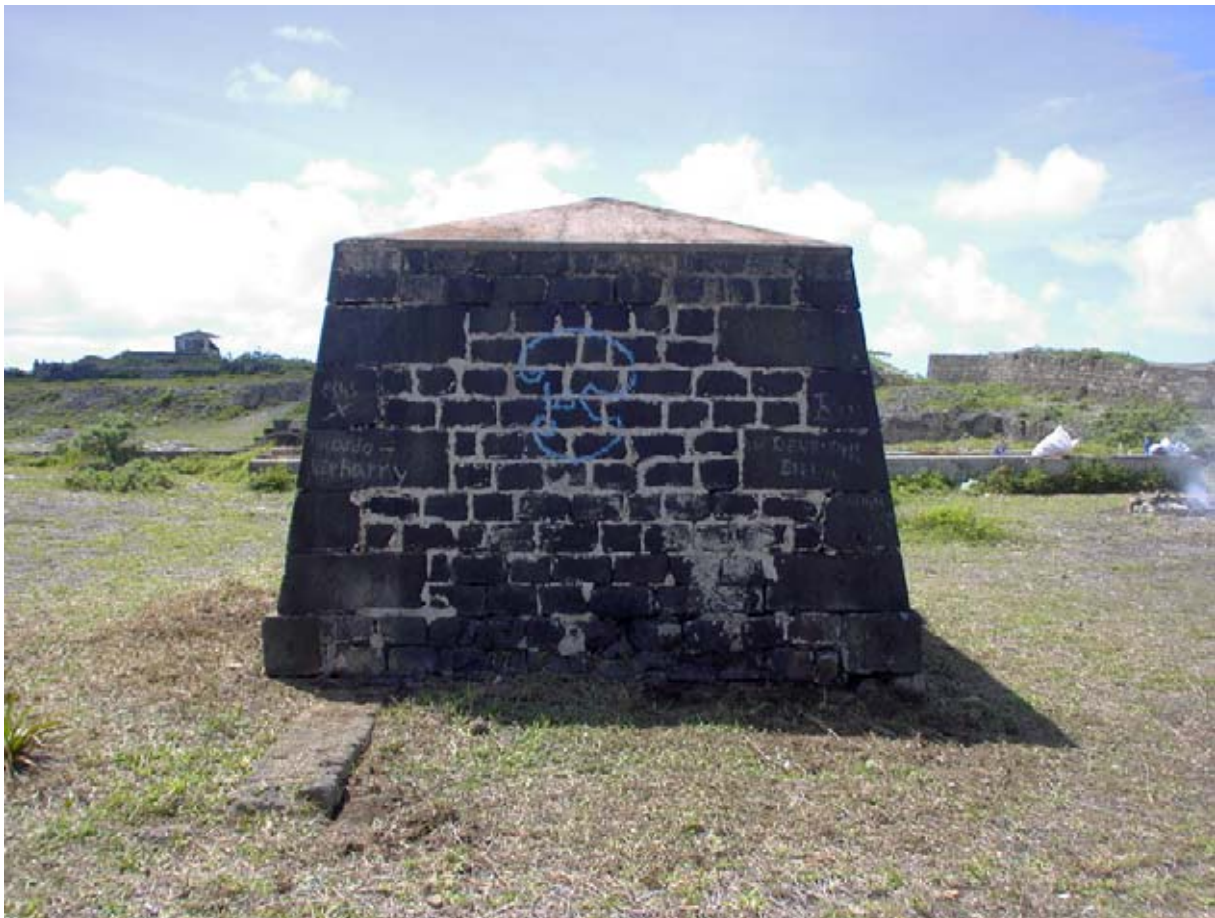
Coral walling projecting from beneath the Shot Furnace. (02jv1102)
