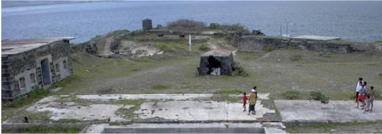
The Barracks (Structure 5) with Structure 18 at right and part of the cistern in front. (02jv0318)
