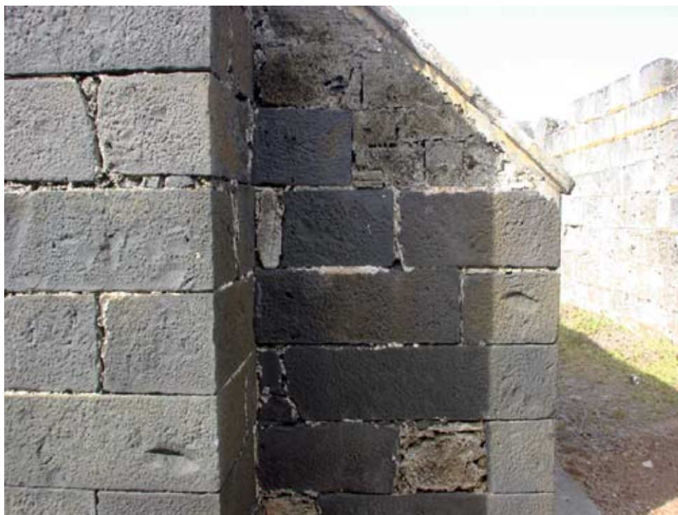
Basalt and coral construction showing the coral roof slates. (01jv0416)
