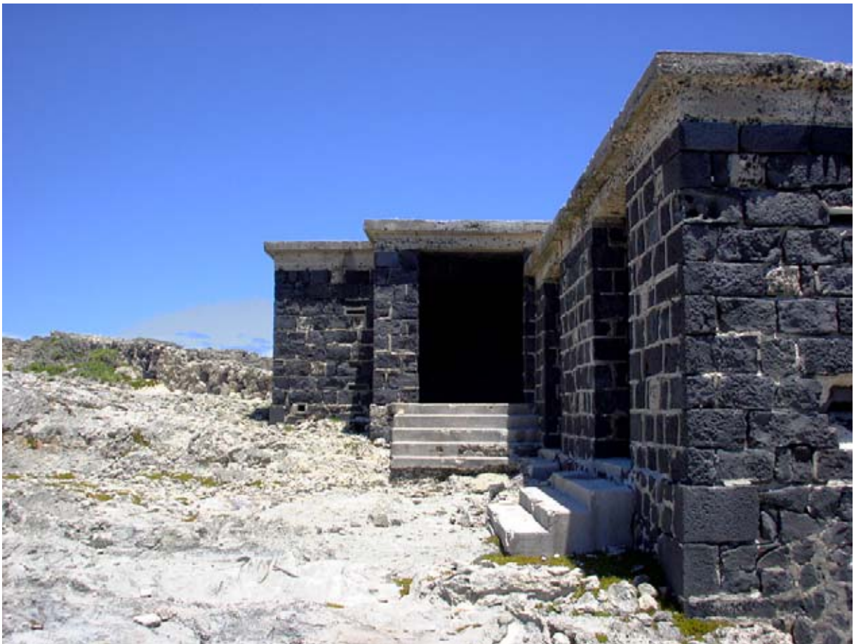
The Western, Searchlight, Building from the north-west. The WW II concrete steps were made in situ. (02jv2114)
