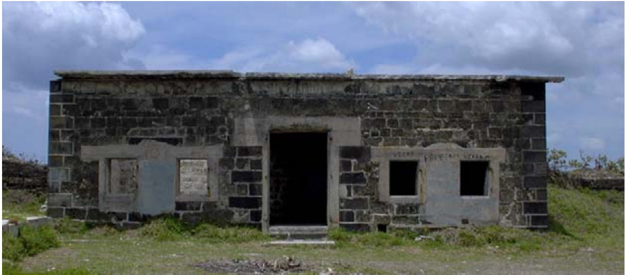
The Storehouse Generator Building showing WW II modifications to the façade that entailed raising the door and replacing single windows with pairs in such a way that there was a new window in front of each generator. The basalt lintels to the original French windows can be seen. A new reinforced concrete roof was added and four openings were made at the level of the electric cable ducts in the new floor, one of which can be seen to the right of the door below the corner of the window. (02jv0114)
