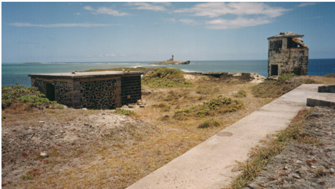
The Upper Battery with Observation Tower and the Central Building which formed part of an aiming system in WW II. The concrete platform links the two horseshoe-shaped gun emplacements, of which part of the southernmost can be seen. The stones just visible to the immediate right of the concrete are the facing of the earlier French battery. (01cn0131)
