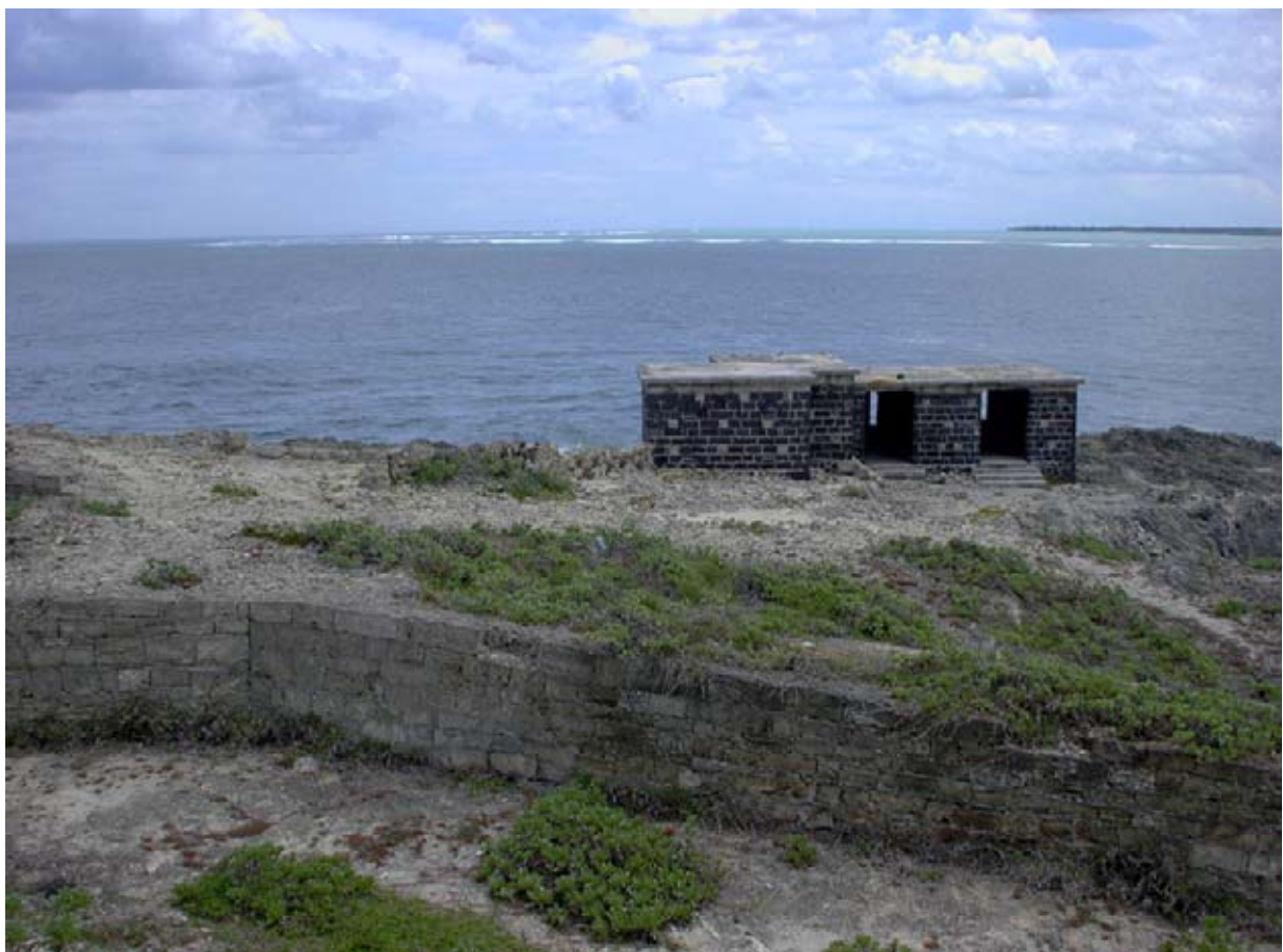
The Western, Searchlight, Building - Structure 12 - showing its commanding position covering the pass. (02jv0310)
