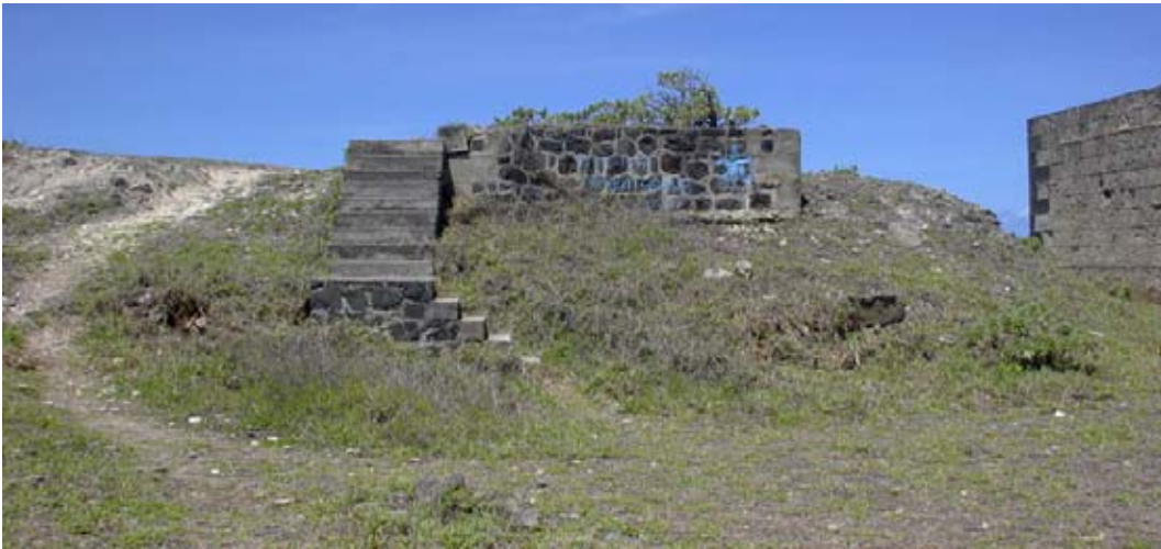
The steps leading up to Structure 20. (02jv1320)
