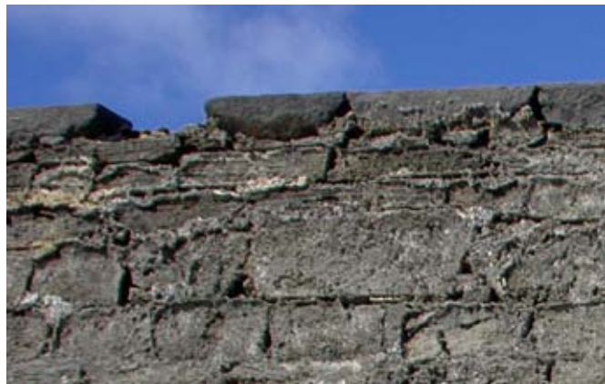
Basalt coping stones on wall B. (m02jv1702)
