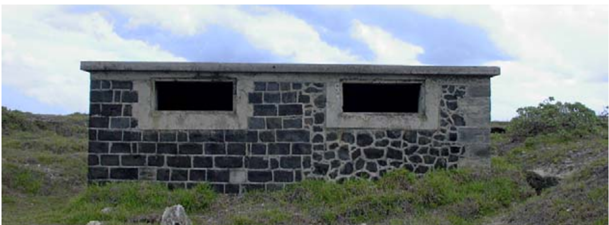
The east side of the Central Building showing the additional room, in a different style, on the right and the two large WW II windows. (02jv0404)
