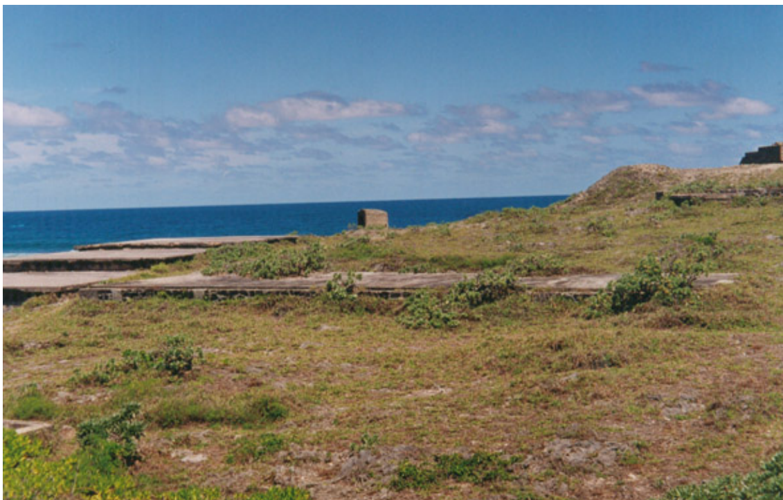
Structure 28 with the Underground Generator Halls at left and the East Sentry Post at centre. (02cn0413)
