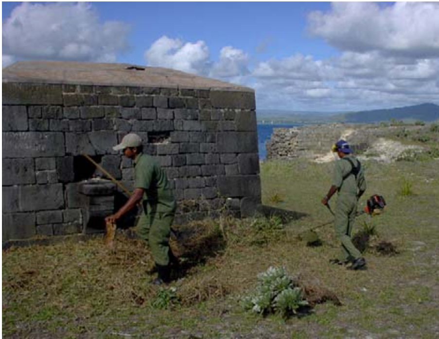
Cutting back the vegetation around the Shot Furnace. (02jv1022)
