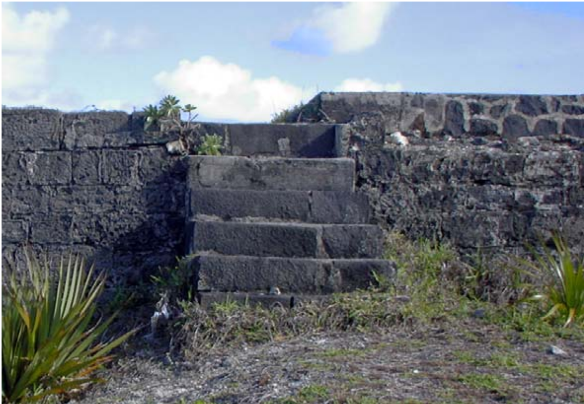
Staircase leading on to the Structure 22. (02jv1015)
