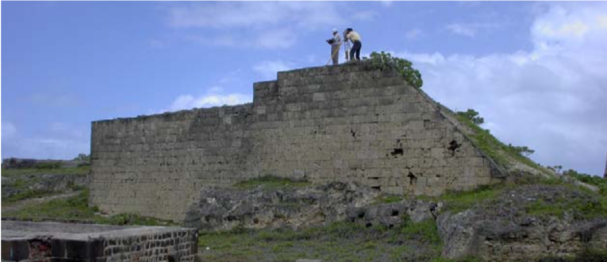
The North Wall and Rampart of the Upper Battery. The angle of slope is 45°, the berm (missing two top stones at left) is 6.00m wide and the terrace 10.0m. (02jv0612)
