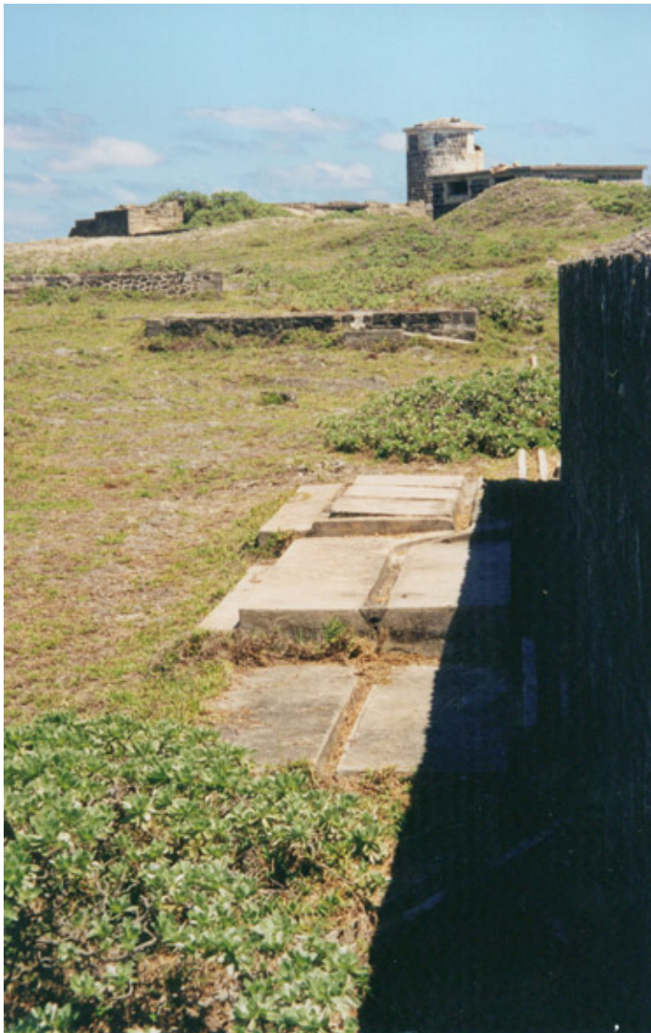
Structure 26, looking towards Structure 16, showing how the drain from the kitchen served both buildings. (02cn0414)
