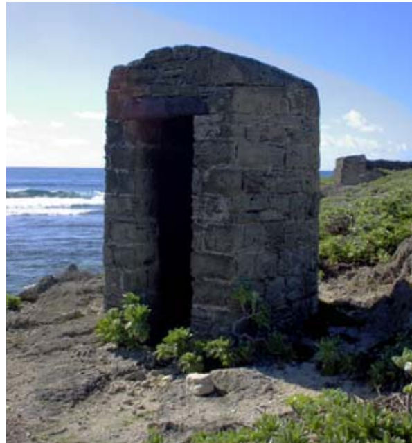
The East Sentry Post founded on bedrock. (02jv1605)
