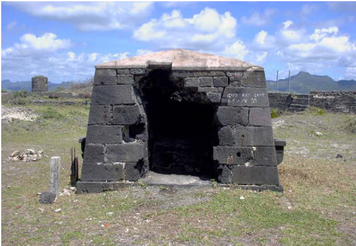
The front and east side of the Shot Furnace with a fragment of an earlier structure at the front right. Note the opening at the front of the roof, the single course of offset footings and the drafted margins of the basalt ashlar. (02jv1023.
