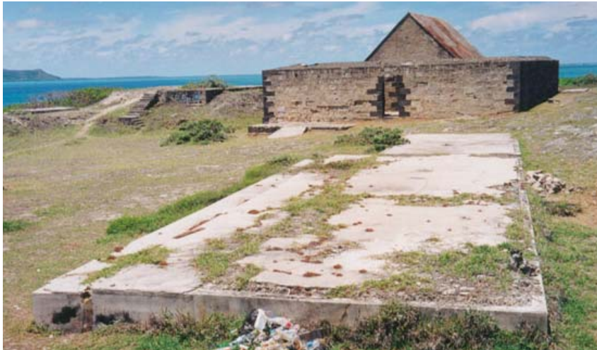
Later Barracks (Structure 6) were built over the French Barracks. (m02jv0402)
