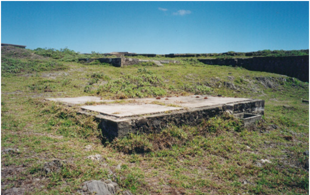
Kitchen (Structure 16), showing the sump for the drain, with Structure 14 behind. (02cn0418)
