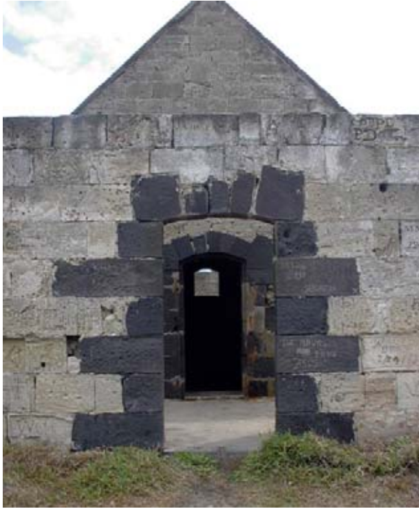
The axial alignment of the enclosure wall and powder house doors and the rear window. Note the low arches and WW II concrete surface. (01jv0620)
