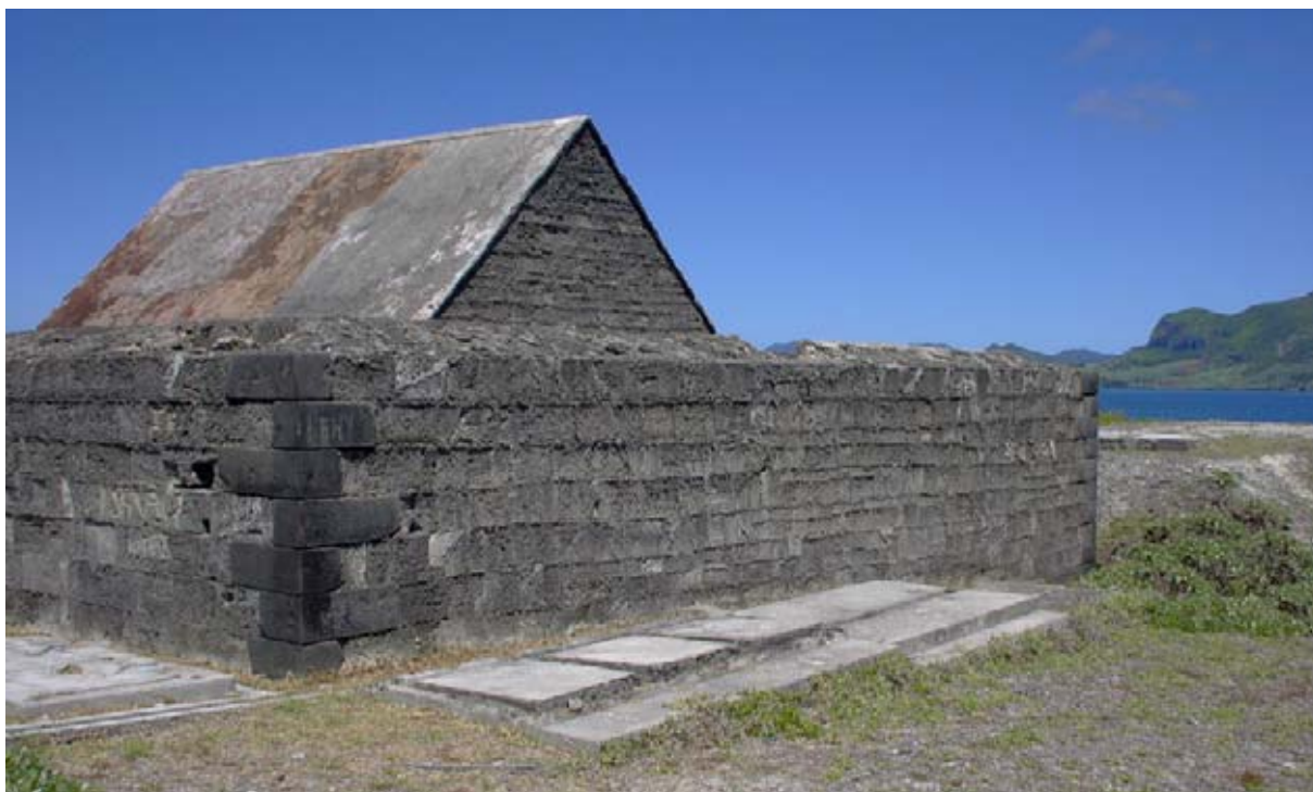
Washing Facilities, Structure 26, by the east wall of the Powder House Enclosure. (02jv2207)
