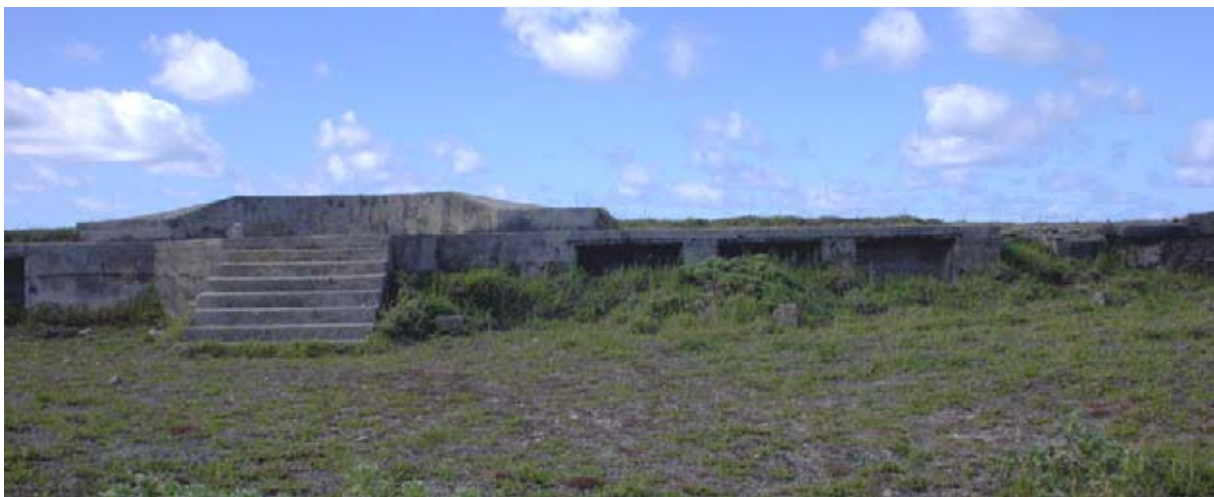
The northern gun emplacement and steps with shell cabins to the right. (02jv2016)
