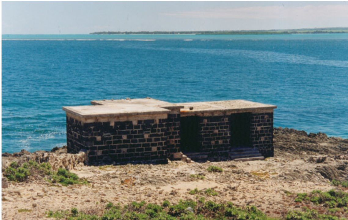
The Western or Searchlight Building, Structure 12. (02cn0427)
