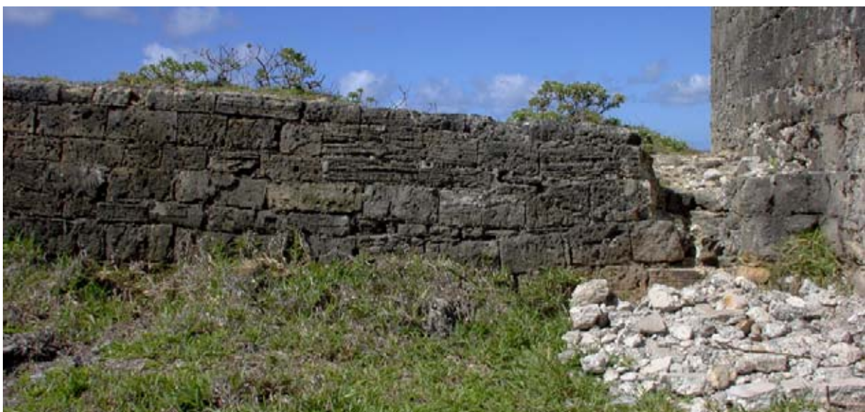
The junction of Wall E and the Storehouse (Structure 2). The two walls are bonded together but camp fires that have been frequently lit in the corner over recent years have caused serious deterioration of the stone. (02jv1924)
