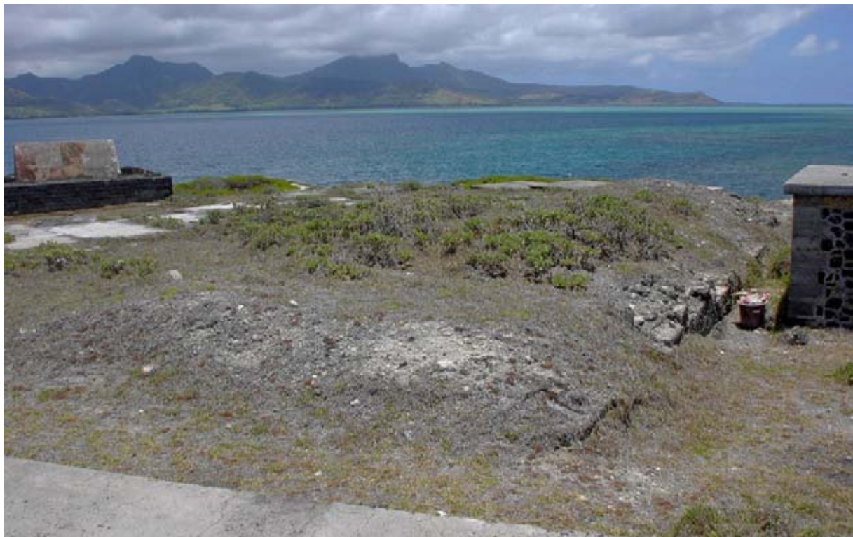
The Platform of Structure 13 from the Upper Battery with the Central Building at right and the roofing of the Underground Generator Halls beyond. (01jv0204)
