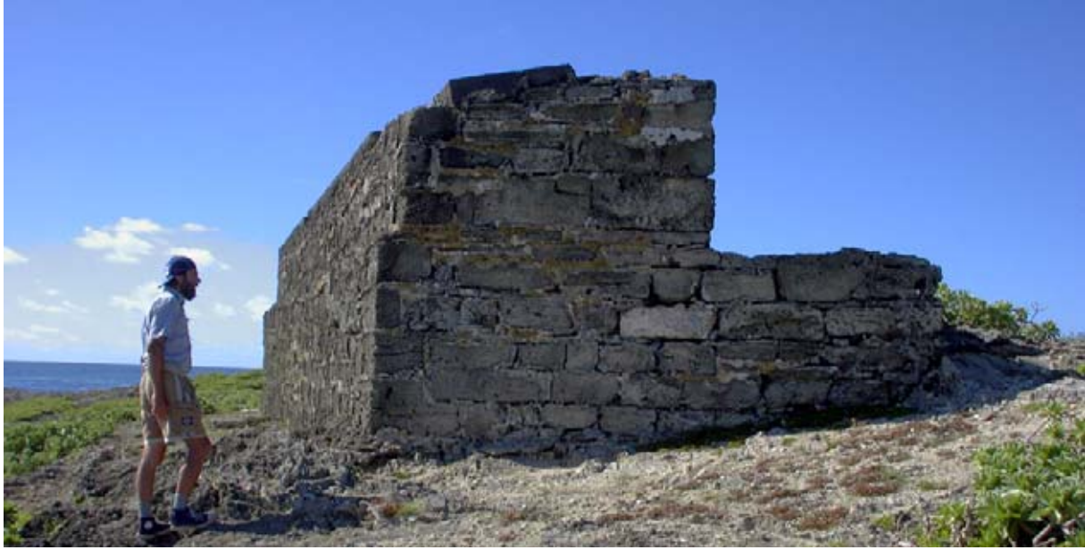
The end of Wall B showing the sloping top edged with basalt coping-stones, the offset and the low return terrace wall. (02jv1618)
