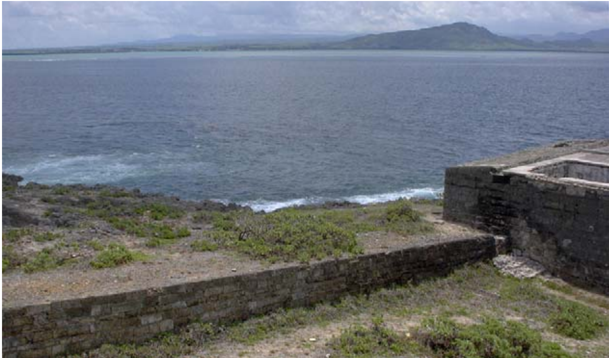
Wall E with the berm and bank beyond. (02jv0312)
