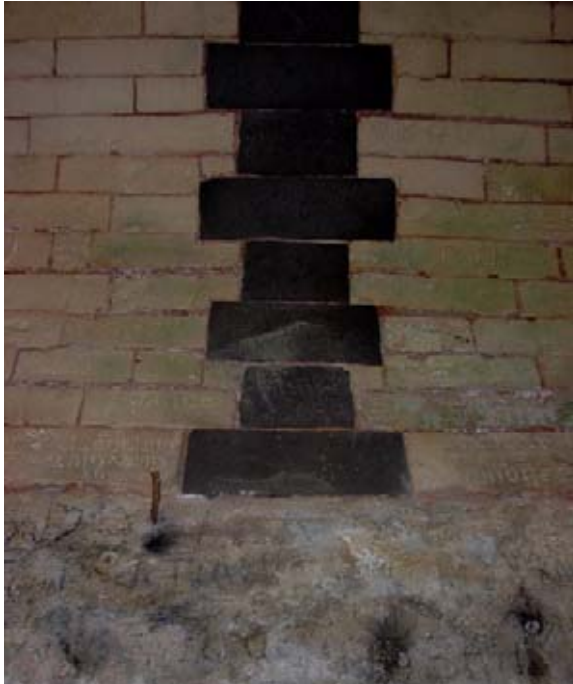
Details of the barrel vaulted ceiling showing the two sides of a basalt arch, the cutting of the fossilised coral blocks to fit and support the basalt during construction, and the use of waterproof lime mortar mixed with crushed brick for the vault. Some of the graffiti carved into the coral by British soldiers in the 1840s are visible. The walls are rendered below the springing. (01jv0601 & 0602)
