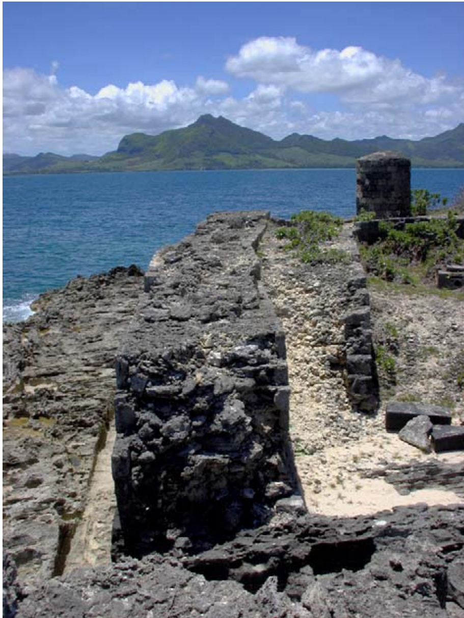
The North-Western Platform looking north from the breach in Wall F. The rock-cut trench for the Buttress is at left. The face stones and mortared rubble core of Wall F can be seen. The loose rubble fill of the ramp platform retained by, Wall G runs beneath the North-West Sentry Post. 02jv1212)
