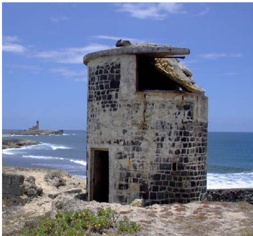
The Observation Tower with WW II blocking below the wide window. (01jv0203)
