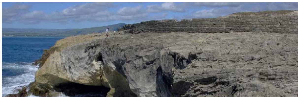
The main sweep of the Lower Battery (Wall A) from the south-eastern spur of the island. The top of the battery wall was originally higher, but it was demolished to the base of the cannon emplacements when the Upper Battery was constructed. (02jv1806)
