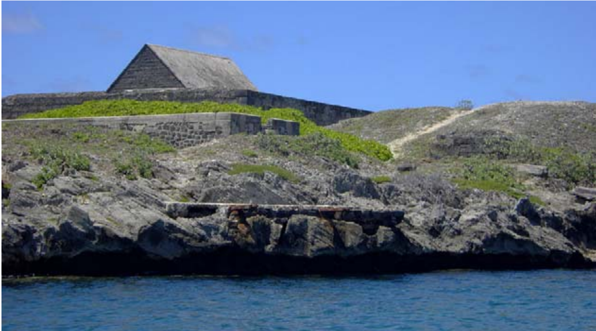
The cuttings in the rock below the World War II toilets (Structure 30) taken from the sea at low tide. The concrete platform and iron rails rest on an earlier rock-cut platform. (02jv1515)
