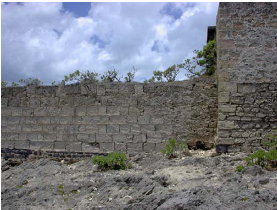
The end of Wall F was broken where the ashlar face stones step down, and it was rebuilt when the Storehouse was constructed. The bushes are growing on the high bank behind the wall. (02jv0201)
