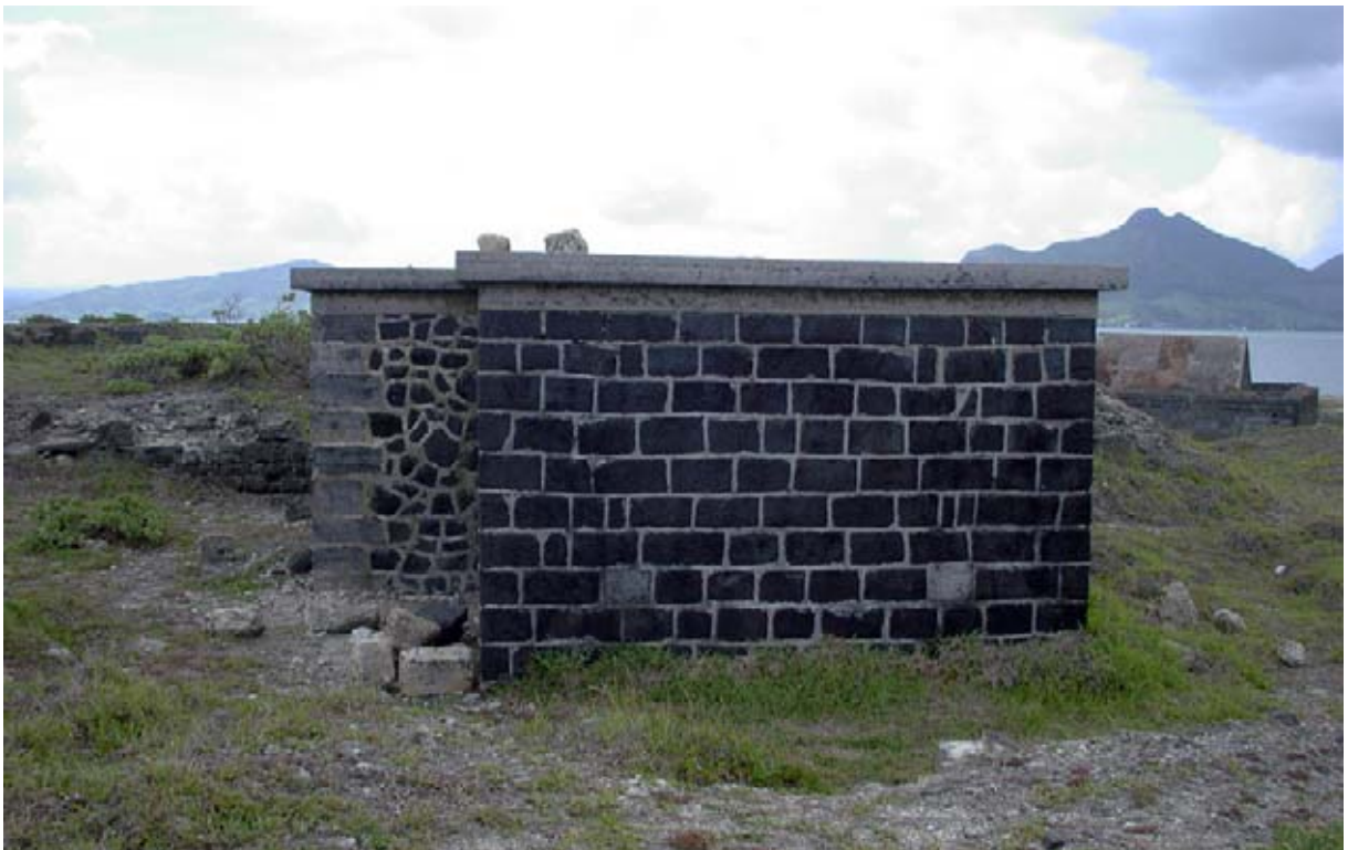
The south side of the Central Building. (02jv0403)
