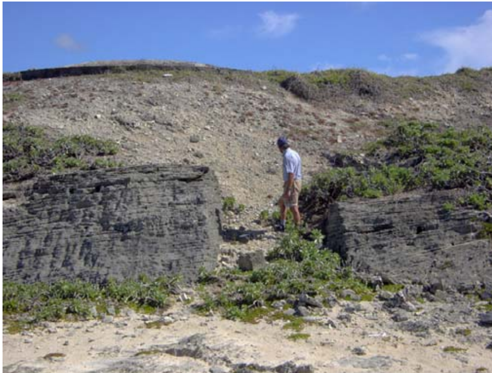
The cutting, now partially filled by the rampart of the Upper Battery that may perhaps be the end of the passage shown on Map 1. (02jv1901)
