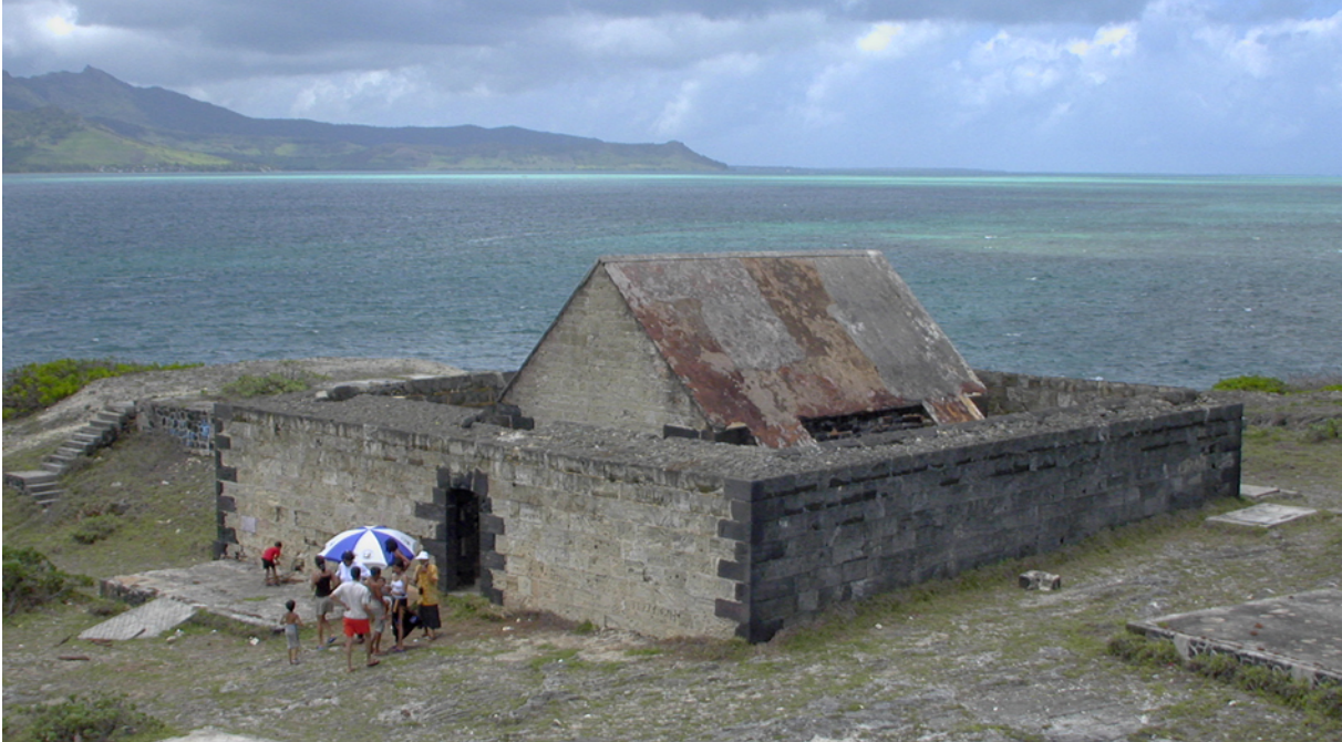
The Powder House, Structure 1, as seen from the Upper Battery. (02jv0316)
