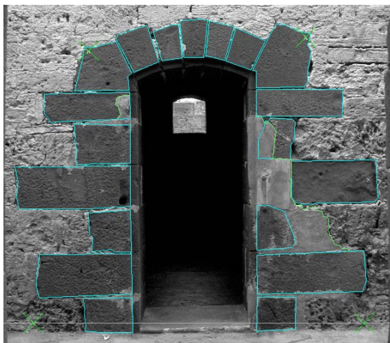
Rectified photo of entrance door to vaulted room imported into AutoCAD with digitised drawing of basalt blocks superimposed. (Not printed to scale)
