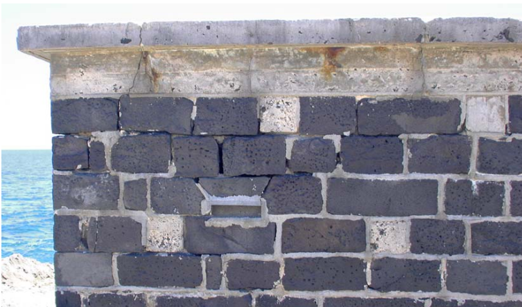
Concrete tie blocks and inclined vent.
