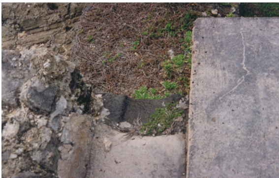
Northern part of roof showing rubble core of back wall and gutter between original back wall and WW II concrete roof. (02cn0104)
