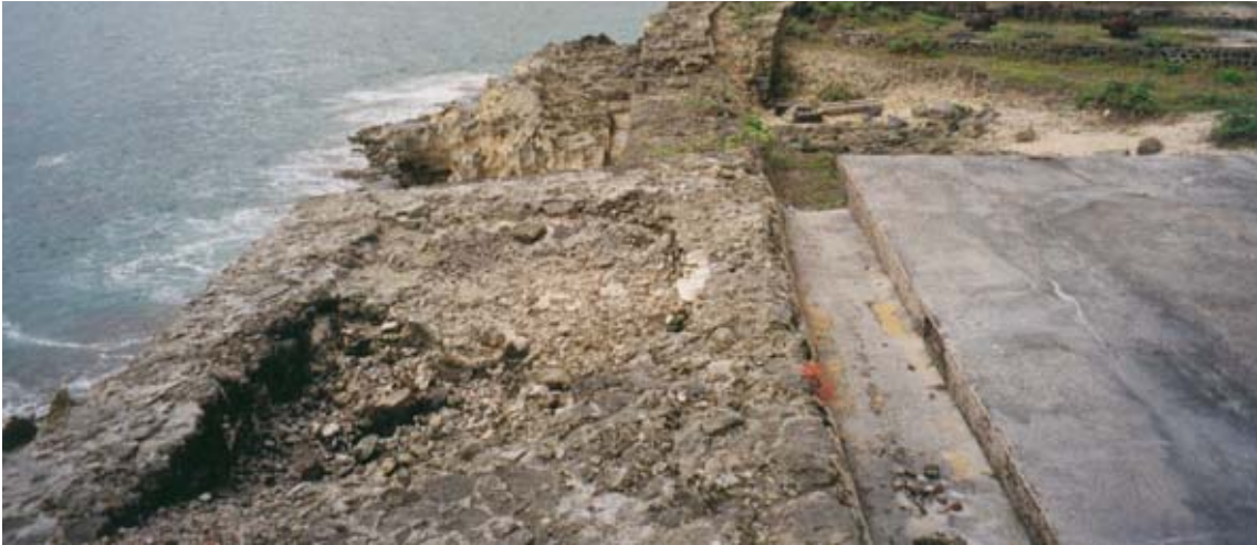
Northern part of roof showing rubble core of back wall and gutter between original back wall and WW II concrete roof. (02cn0104)
