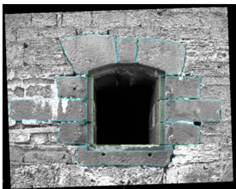
Rectified photo of rear window to vaulted room imported into AutoCAD with digitised drawing of basalt blocks superimposed. (Not printed to scale)
