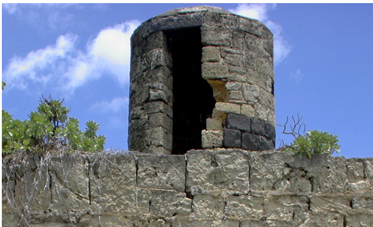
The North-West Sentry Post built on top of the North West Defences. (02jv0217)
