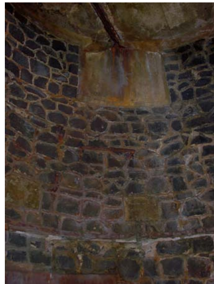
Traces of first floor timbers, blocked window and iron beam. (02jv0915)
