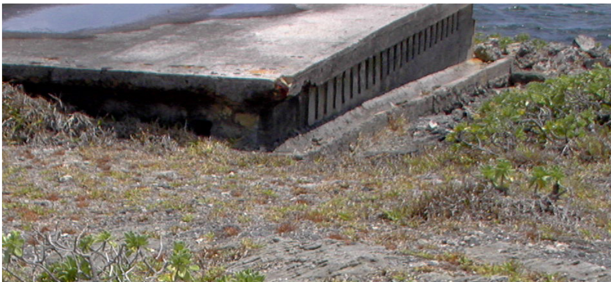
Concrete drain and vents under the southernmost roof slab. (01jv0115)
