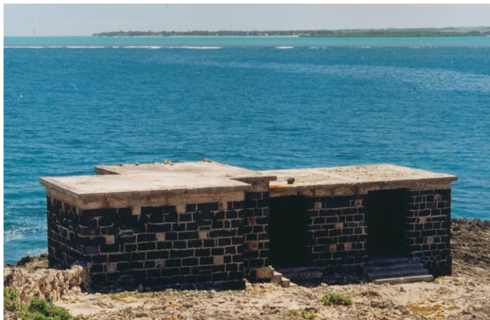
The Western or Searchlight Building overlooking the pass. (02cn0427)
