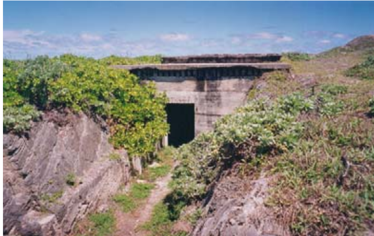
The Underground Generator Halls. (m02cn0417)
