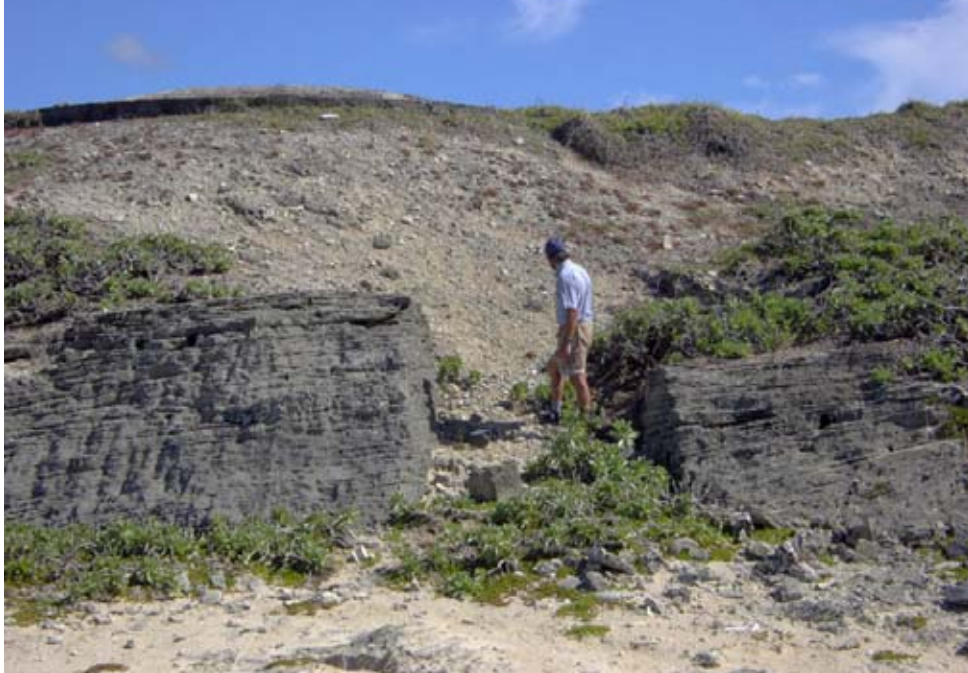
A cutting in the rock on the outer side of the Upper Battery. One of the two Second World War concrete gun emplacements can be seen above the rubble fill makeup of the French rampart. It appears possible that the cutting is the end of a passage that gave level access from the Landing Point and the main structures to the Lower Battery. This hypothesis could be tested by excavation. (02jv1901)
