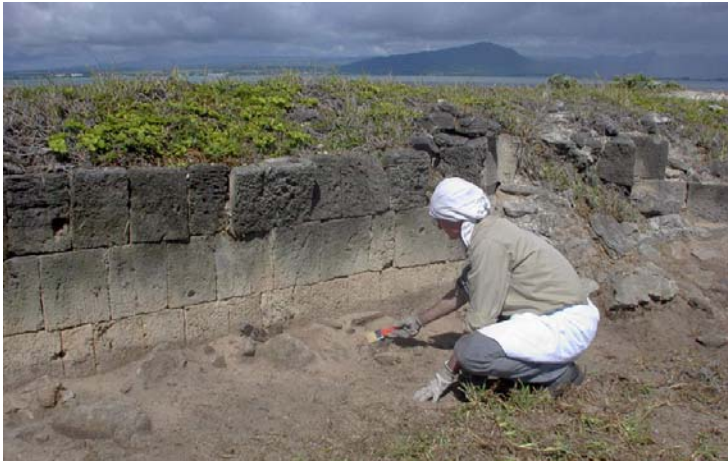
Bradley using a brush in preparation for photography of the Upper Battery parapet. (03jv0205)
