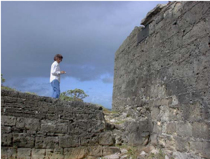
Fay recording graffiti on the Storehouse. (03jv2003)
