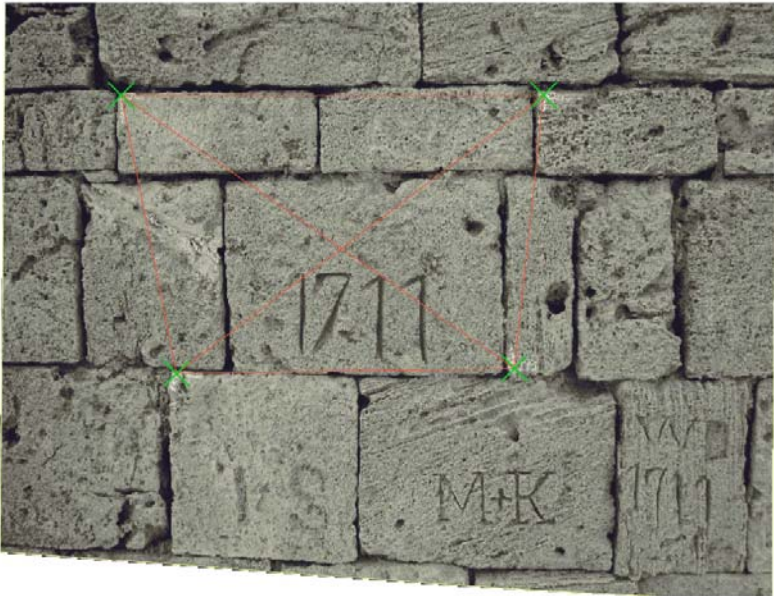
The NW end wall of the Upper Battered reconstituted from a mosaic of rectified photographs for identification of graffiti.
