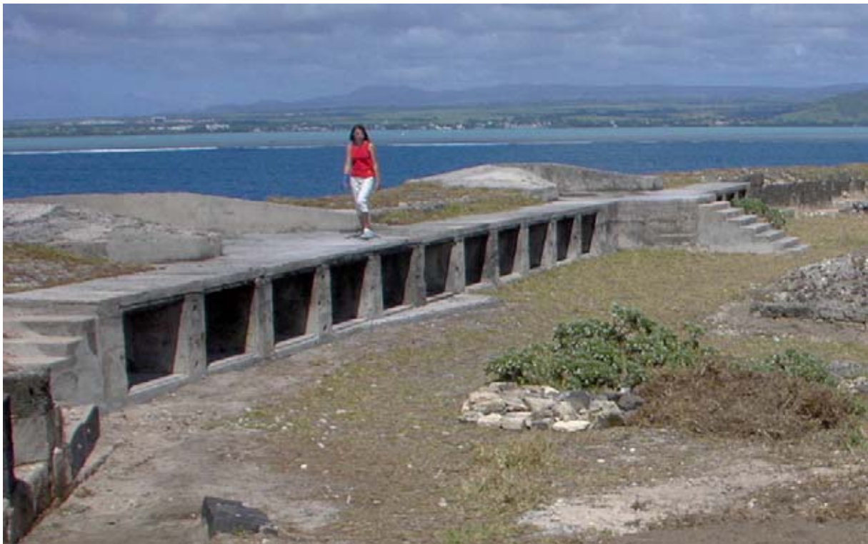
Figure 33: The WWII concrete platform and shell cabins. (03jv3607)
