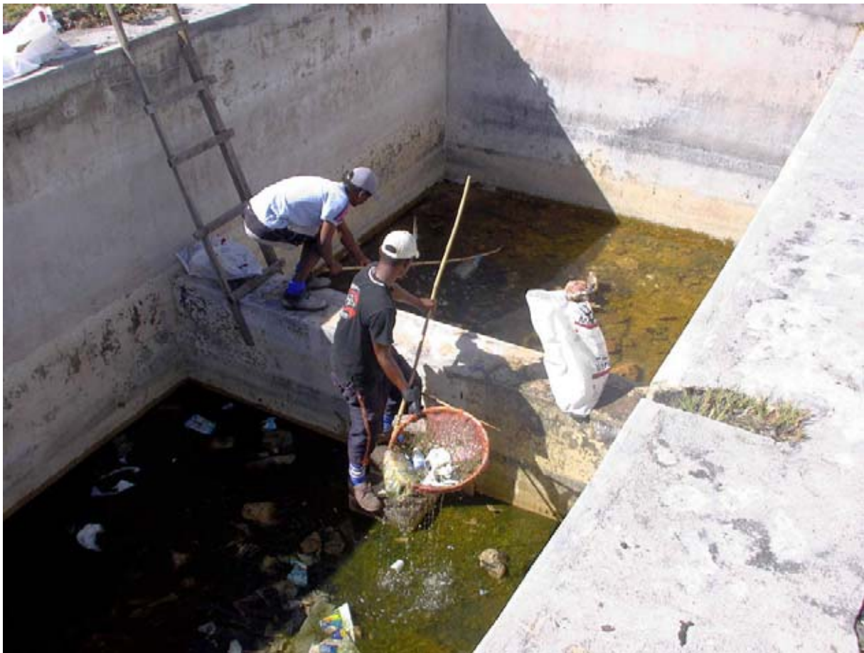
Figure 39: Rubbish being removed from the cistern. (03jv1615)
