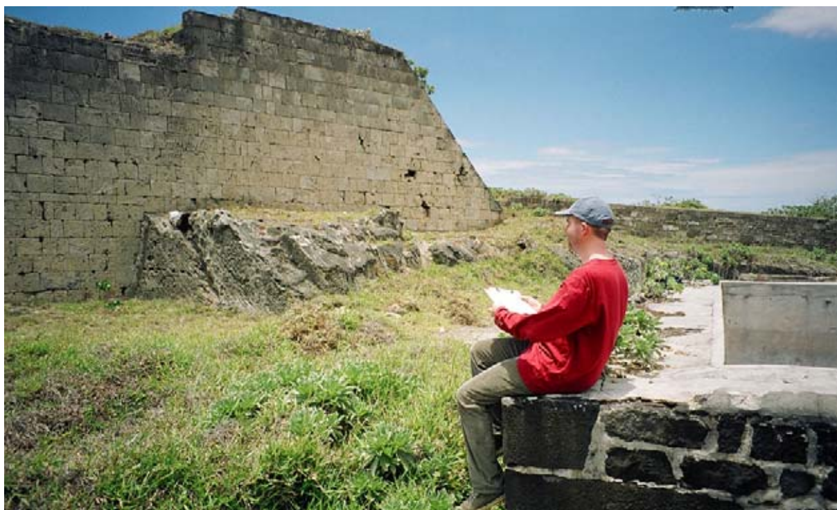
Figure 16: Sketching the north wall of the Upper Battery to note measurements for photo-rectification. (03cn0117)
