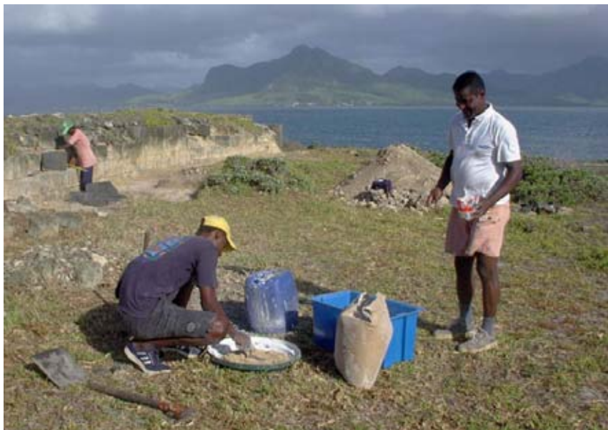
Figure 14: Lime mortar was prepared with 'red earth' brought from the mainland. (03jv1602)
