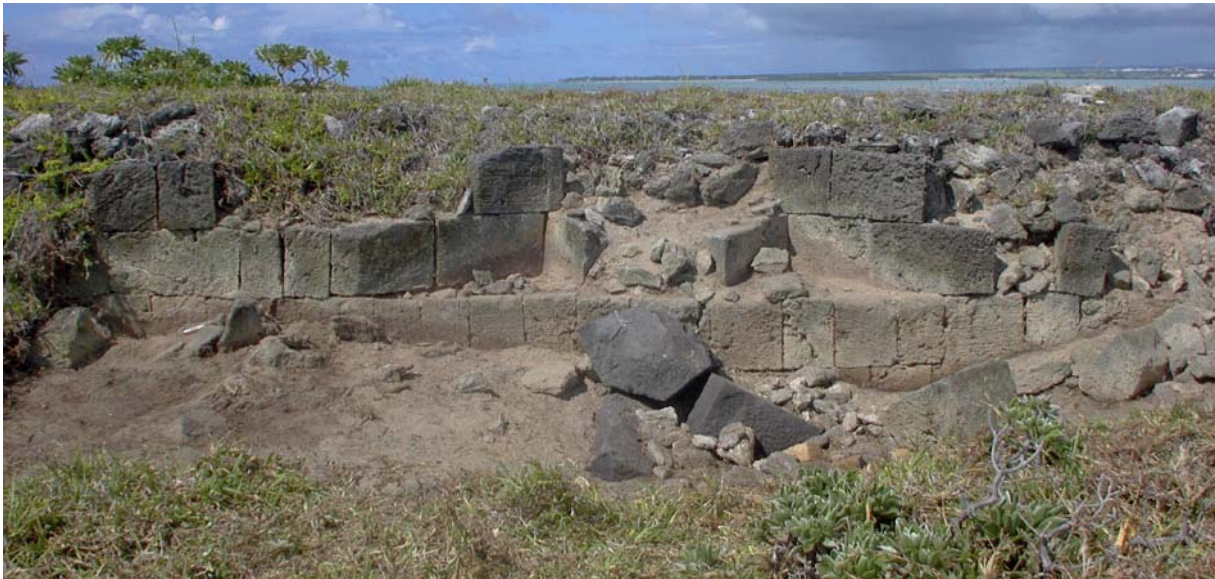
Figure 25: Emplacement 2 after removal of vegetation and before restoration. (03jv0216)
