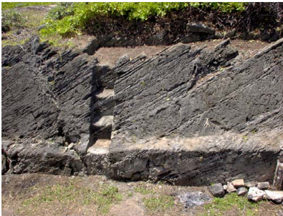
Figure 42: Rock-cut channel and stepped slot, possibly associated with a pre World War II roof. (03jv2903)
