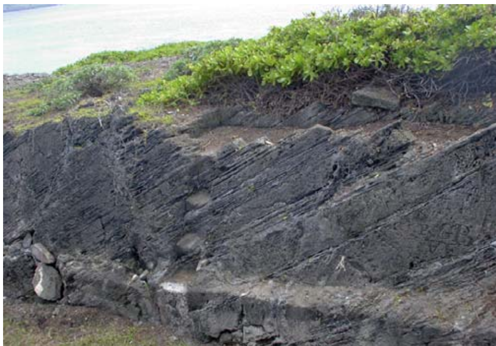
Figure 49: Graffiti were found to be well preserved where protected by overhanging vegetation. (03jv3517)
