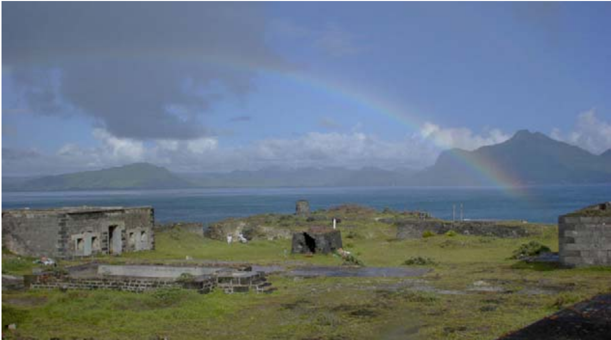
Figure 10: Standing structures are in need of conservation and restoration. (03jv0506)
