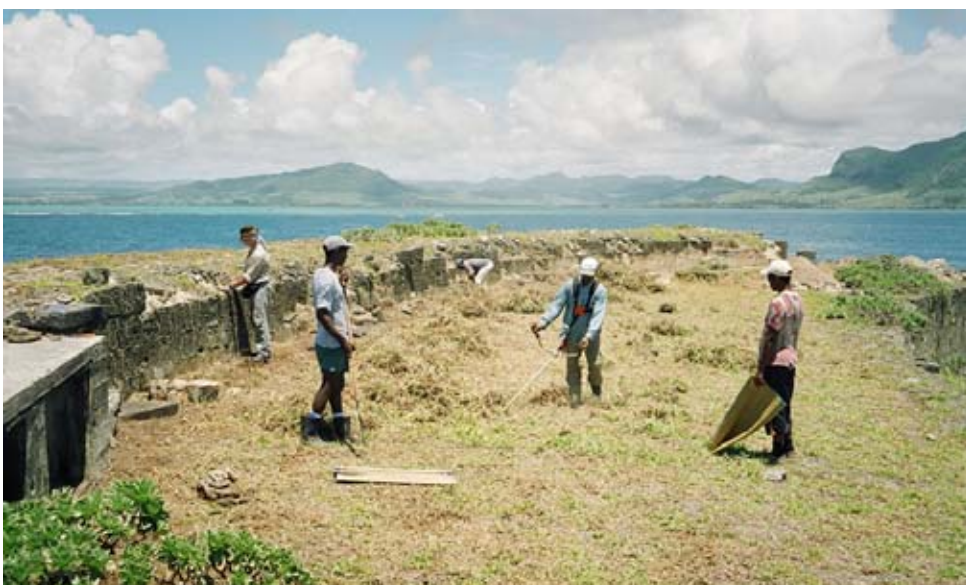
Figure 13: Cutting back vegetation on the Upper Battery. (03cn0134)
