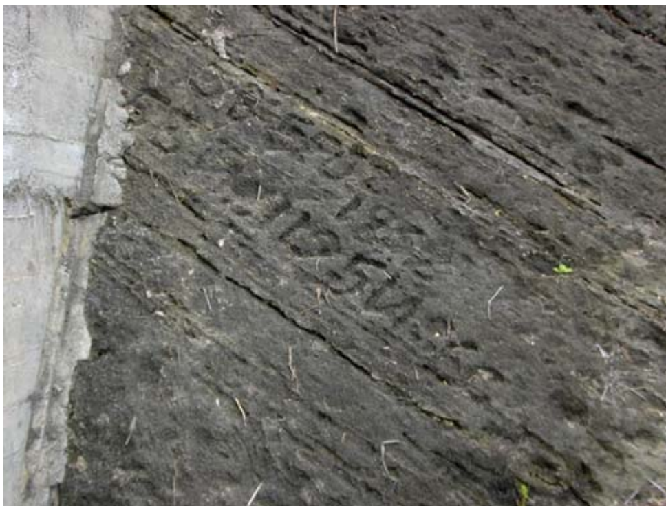
Figure 51: Construction of the World War II Generator Halls, at left, covered many graffiti. (03jv3603)
