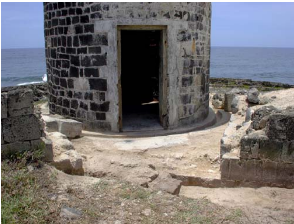
Figure A: Features at the base of the Observation Tower. (03jv1009)
