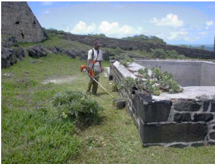
Figure 11. A grass-cutter with nylon line is ideal for cutting back creeping vegetation. (04jv0205)
