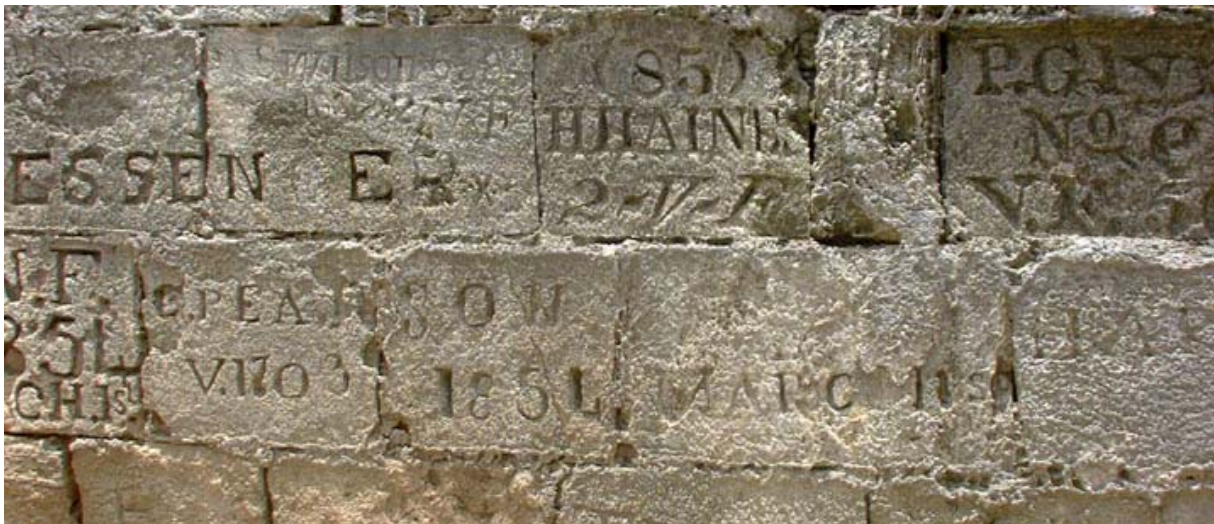
Figure 58. Digital photography produces clear images of graffiti. A scale drawing can be produced from a rectified photo. (04jv0538)
