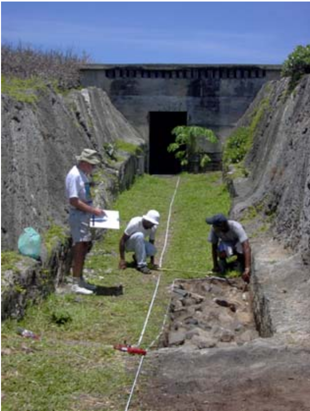
Figure 17. Rudy and Vickram, helped by a workman, drawing the top of the stone fill of trench TR12 in the enigmatic Ditch. The entrance to the Generator Hall can be seen in the background. (04jv2021)
