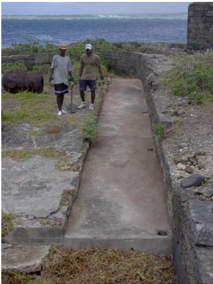
Figure 27. The corridor at the front of Structure 31 built against the earlier Battery wall. Post holes indicate that it was roofed. (04jv1220)
