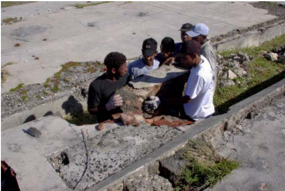
Figure 24. The workmen uniting efforts to put back a large basalt block dislodged from the settling tank of the Cistern. (04jv0905)
