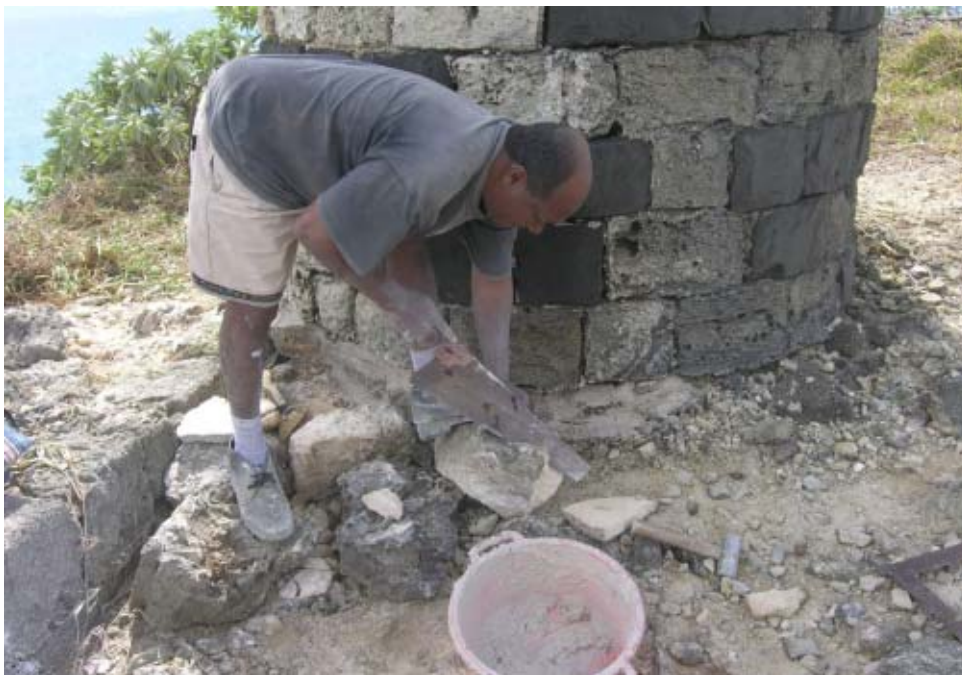
Figure 12. Patrick, a local mason with experience of cutting soft coral in his native Rodrigue, demonstrated that the soft coral could be easily cut and shaped with a saw. (mp05nc1422)
