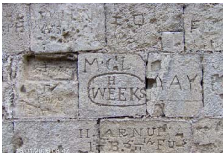
Figure 31. Log put holes for scaffolding, at top right, were first noted while recording graffiti on the walls of the Powder House. (mp06nc0408)
