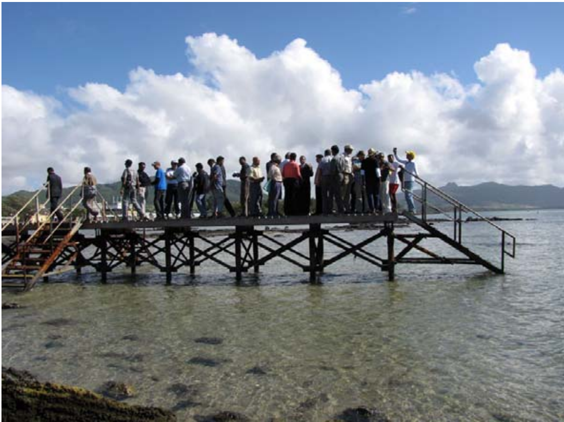
Figure 8. The existing jetty at the Fish Landing Station in August 2009.
